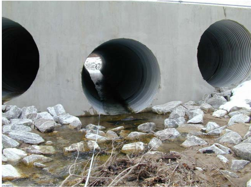
Figure 8 Culvert under Rogers Ave. at Site 228.
