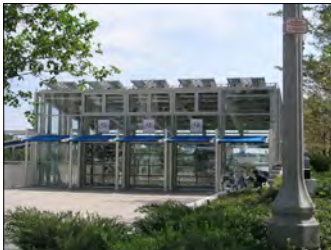
Bicycle Parking Facility
