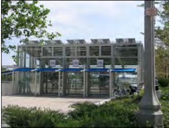
Bicycle Parking Facility
