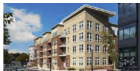
The Arlington Mill Residences on Columbia Pike is a four-story, 122-unit complex that is 100 percent affordable (for 60 percent AMI). It includes 98 two- and three-bedroom units to support larger families and 13 units designated for formerly homeless individuals and families. Image: staff photo.
