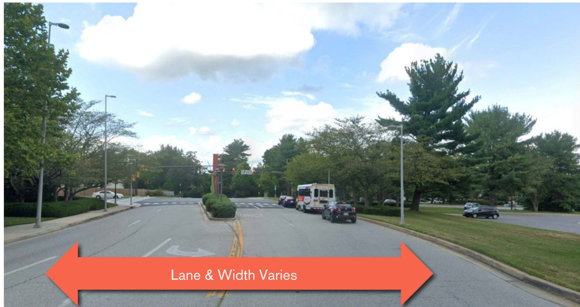
View of Windstream Drive Looking Towards Governor Warfield Parkway
