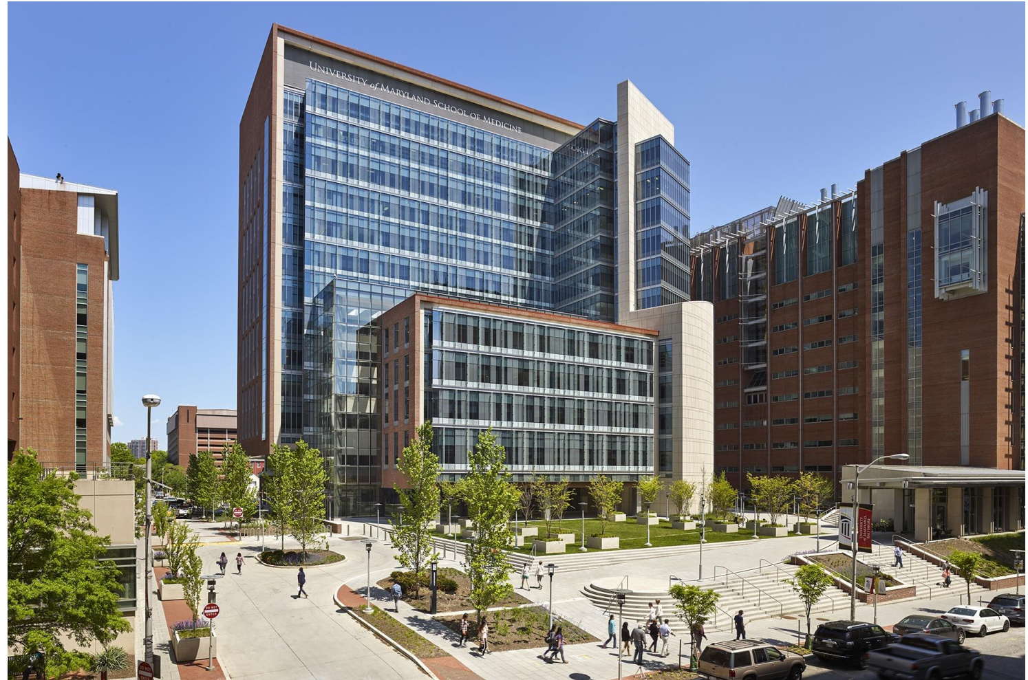
University of Maryland, Health Science Research Facility III (HSRF III)
