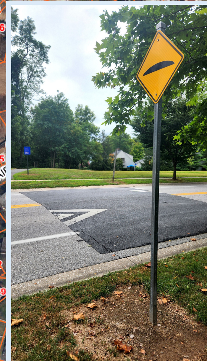
Example of Speed Hump
