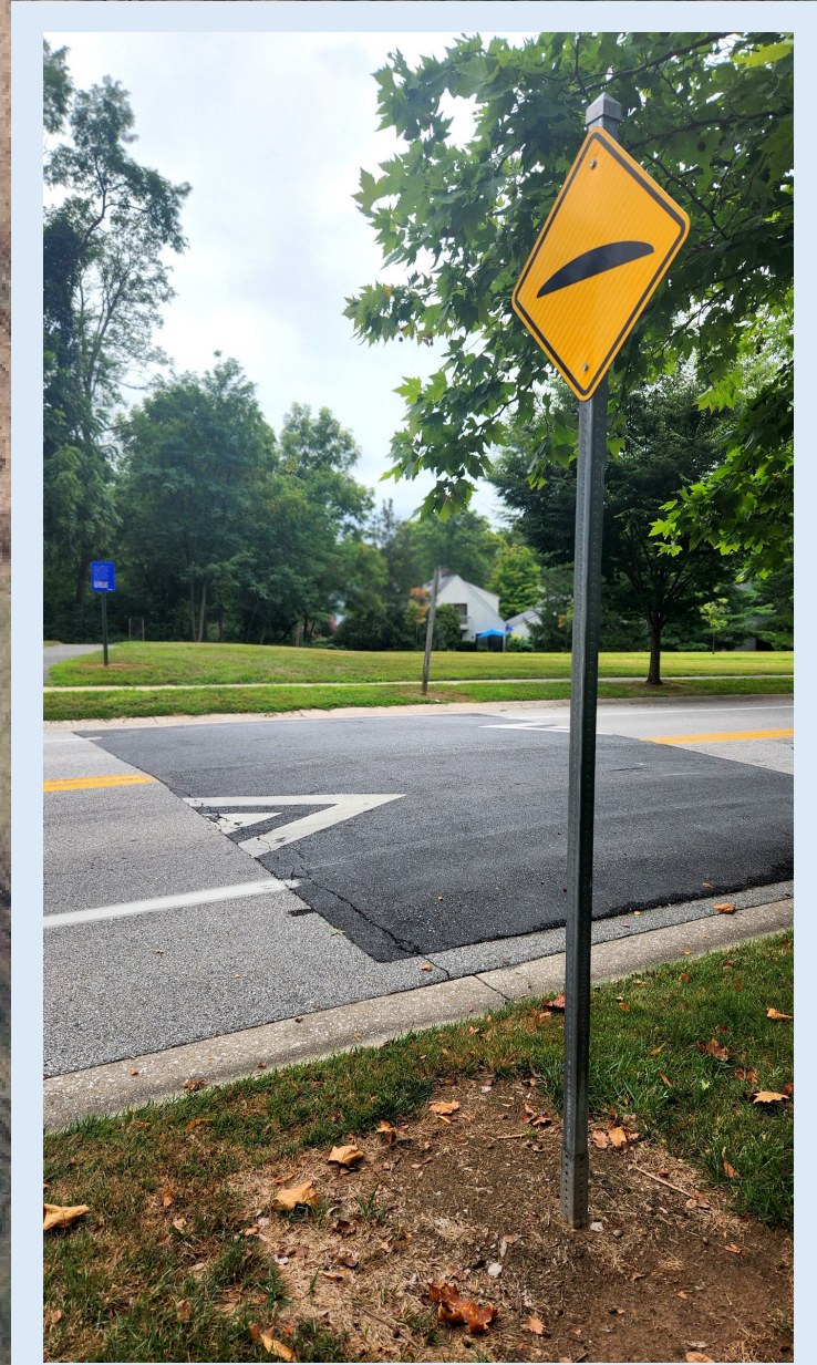
Example of Speed Hump
