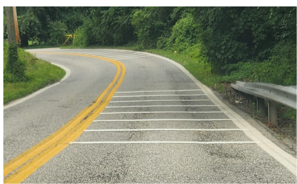
Recently Installed Rumble Strips
