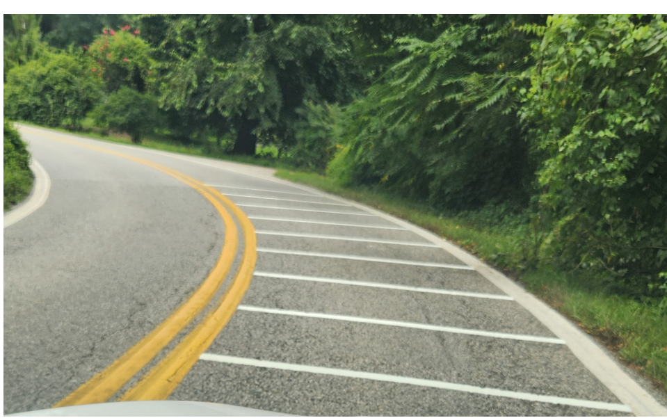
Recently Installed Rumble Strips
