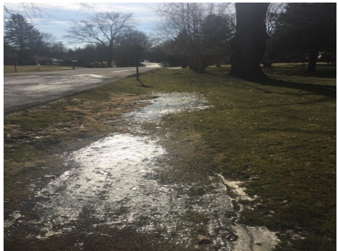
Figure 2: Standing water and erosion in roadside ditch along Greenway Dr.
