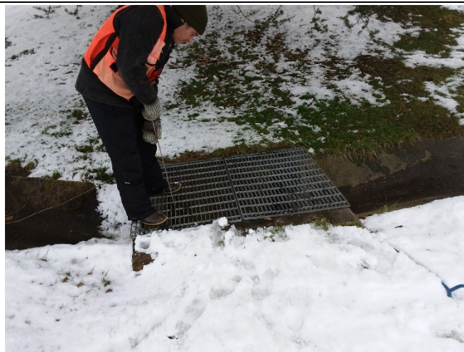
Figure 4: Typical inlet along Spring Meadow Drive.
