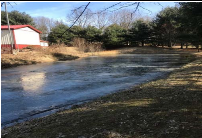
Figure 1: Infiltration facility is filled with standing water.
