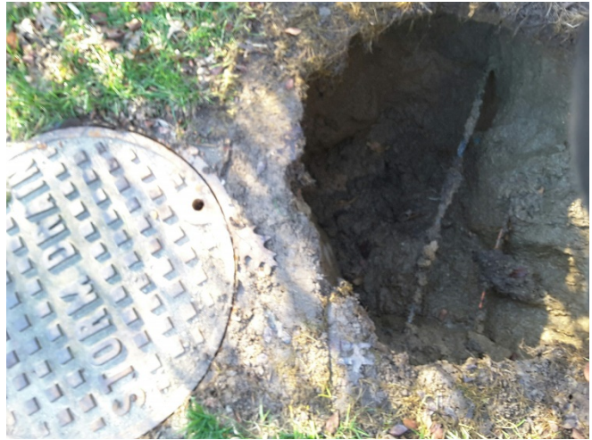
Figure 2: Utilities exposed adjacent to manhole along Dunloggin Road.
