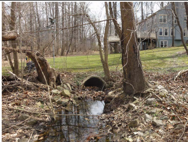
Figure 2: Opportunity to improve existing conveyance system.
