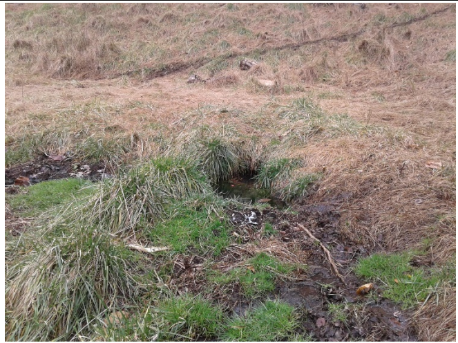
Figure 2: Pond inflow submerged and overgrown.
