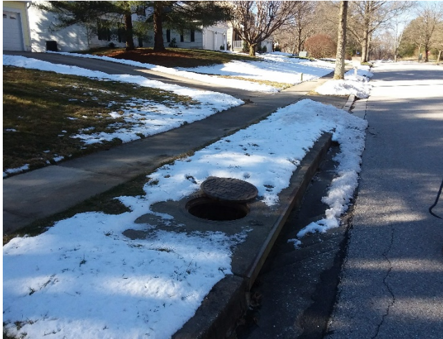
Figure 1: Typical inlet along Sunlit Passage.
