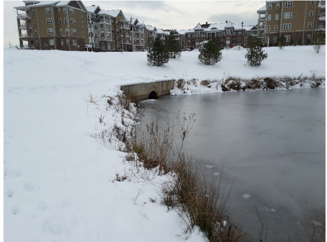
Figure 2: Typical stormwater facility outfall within The Lutheran Village at Miller's Grant development.
