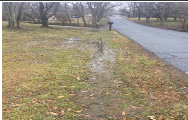
Figure 3: Standing water in ditch along Brookmede Rd.
