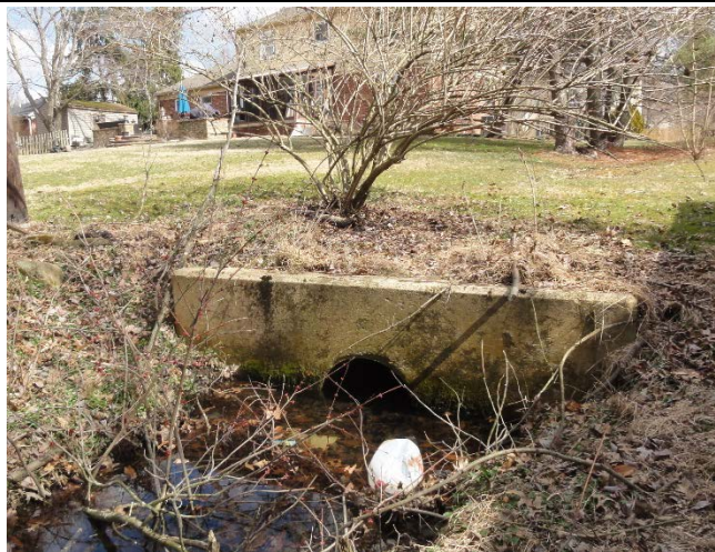
Figure 1: Opportunity to improve existing conveyance system.
