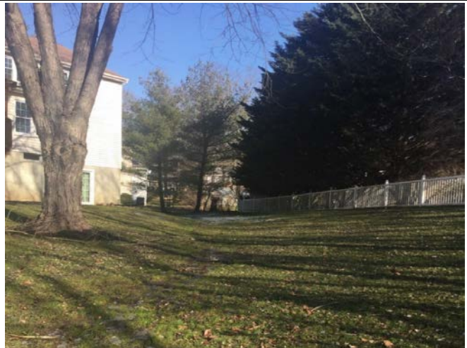
Figure 2: Ponding water behind home at 9543 Michaels Way.
