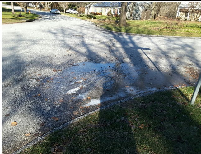
Figure 1: Opportunity to improve existing conveyance system.
