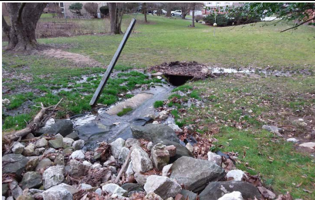
Figure 3: Opportunity to improve existing conveyance system.
