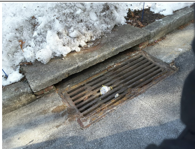
Figure 2: Typical inlet along Plumtree Drive.
