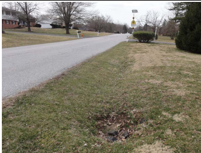
Figure 1: Opportunity to improve existing conveyance system.
