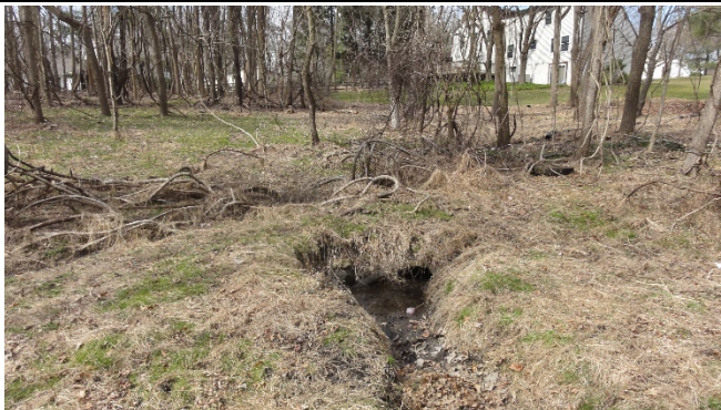
Figure 3: Opportunity to improve existing conveyance system.
