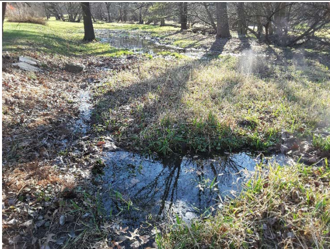
Figure 1: Opportunity to improve existing conveyance system.
