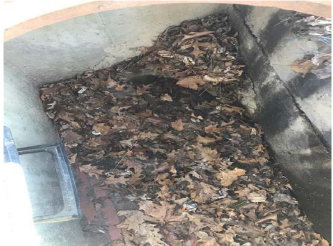
Figure 2: Cleaning recommended inside inlet.
