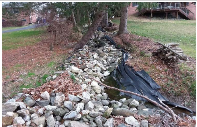
Figure 2: Opportunity to improve existing conveyance system.
