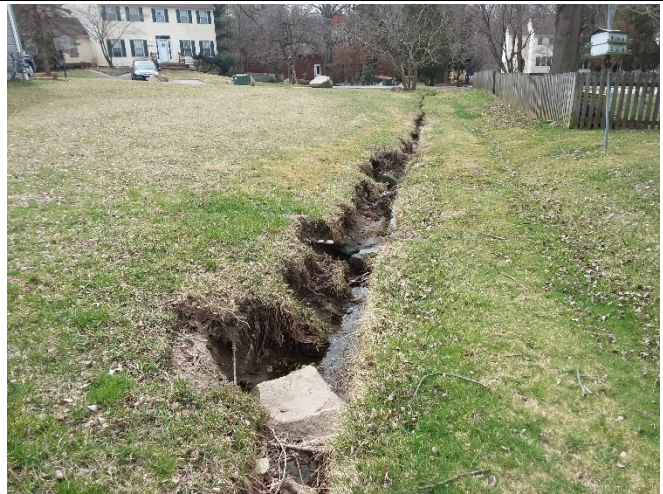
Figure 2: Opportunity to improve existing conveyance system.
