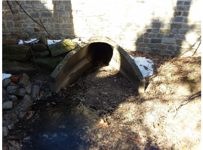
Figure 2: Typical outfall along Bright Bay Way.
