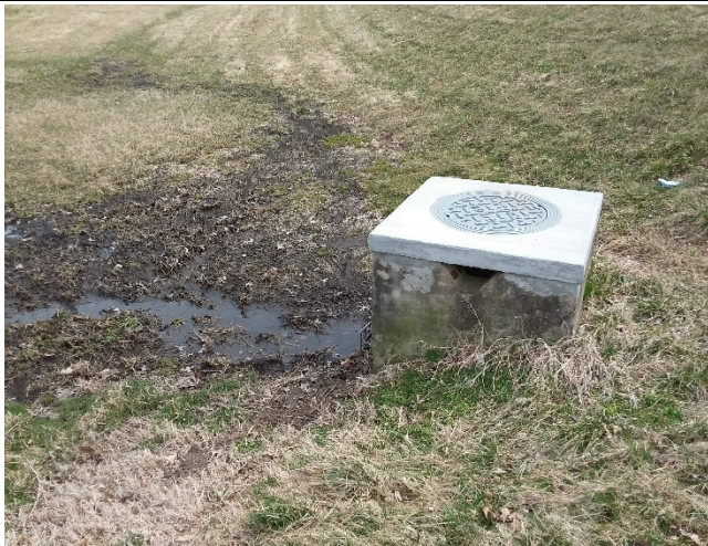
Figure 1: Opportunity to improve existing conveyance system.
