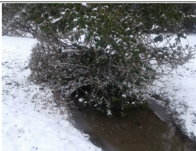
Figure 3: Downstream end of driveway culvert.
