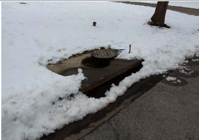
Figure 1: Typical inlet along Gray Rock Drive.
