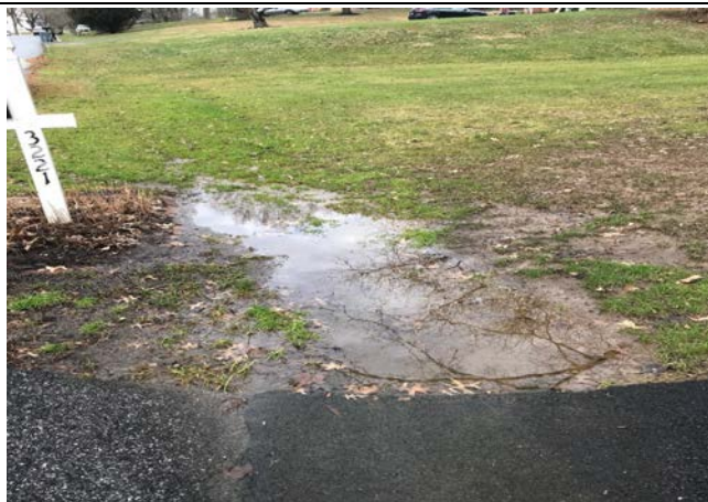
Figure 1: Standing water adjacent to driveway on Hearthstone Rd.
