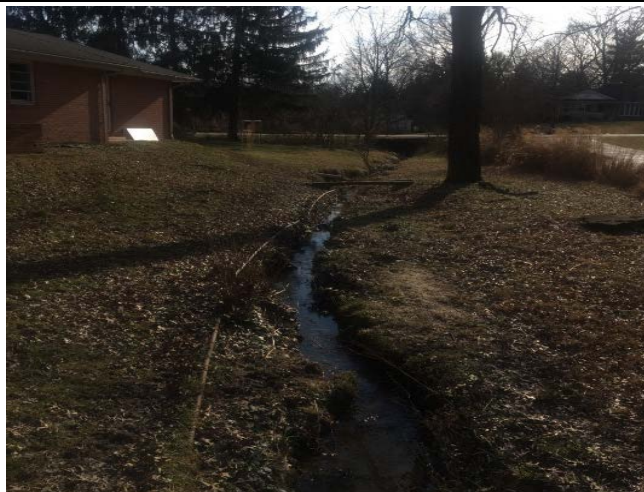
Figure 3: Stream channel upstream of pipe network that is potentially inefficient.
