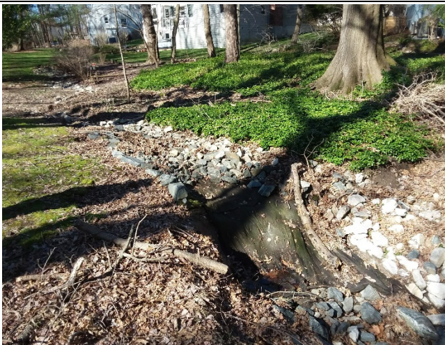
Figure 3: Opportunity to improve existing conveyance system.
