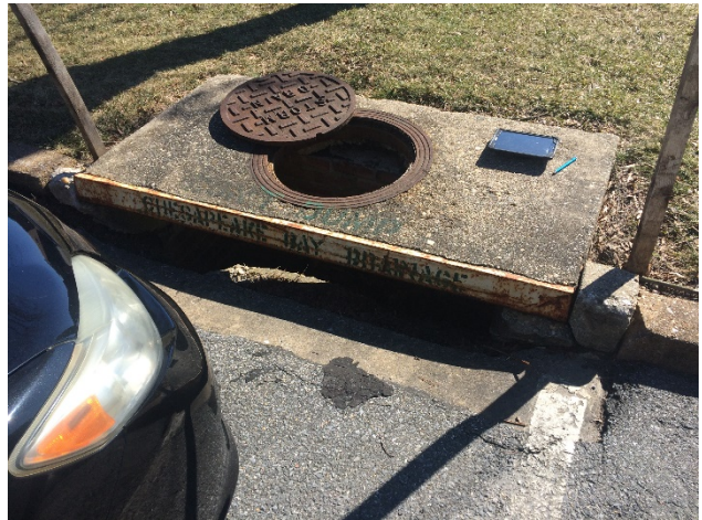
Figure 2: Typical inlet in front of Northfield Elementary School.
