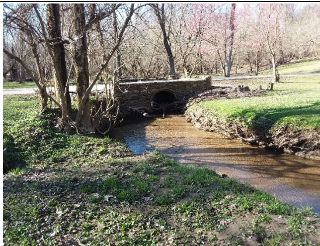
Figure 3: Opportunity to improve existing conveyance system.
