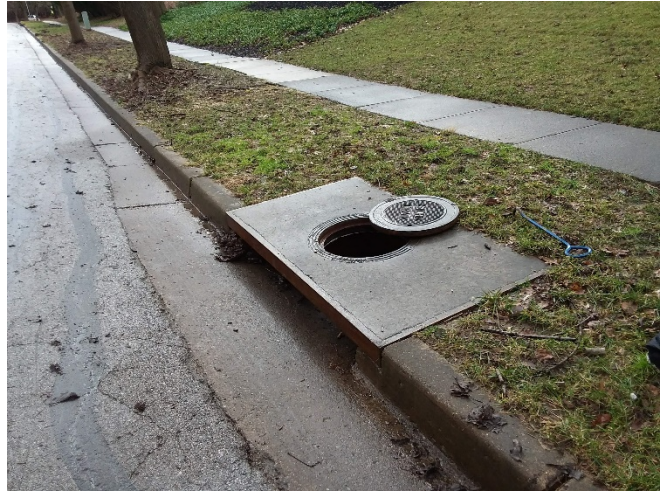
Figure 2: Typical inlet along Firefly Way.
