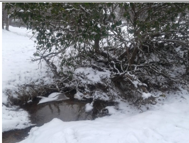
Figure 2: Upstream end of driveway culvert.
