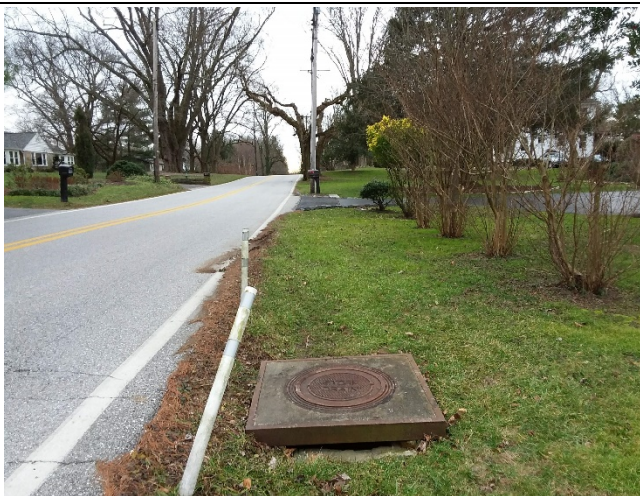
Figure 1: Opportunity to improve existing conveyance system.
