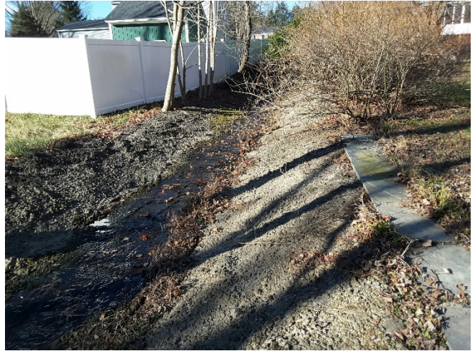
Figure 2: Concrete swale conveying stormwater to Plumtree Branch.
