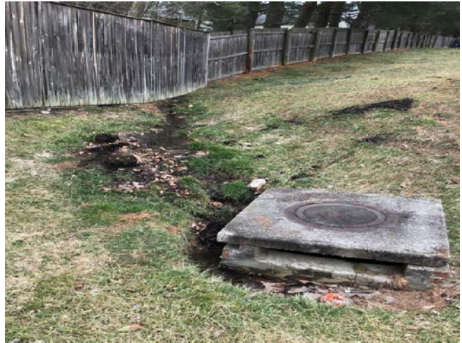
Figure 2: Downstream end of outfall channel leading to inlet.
