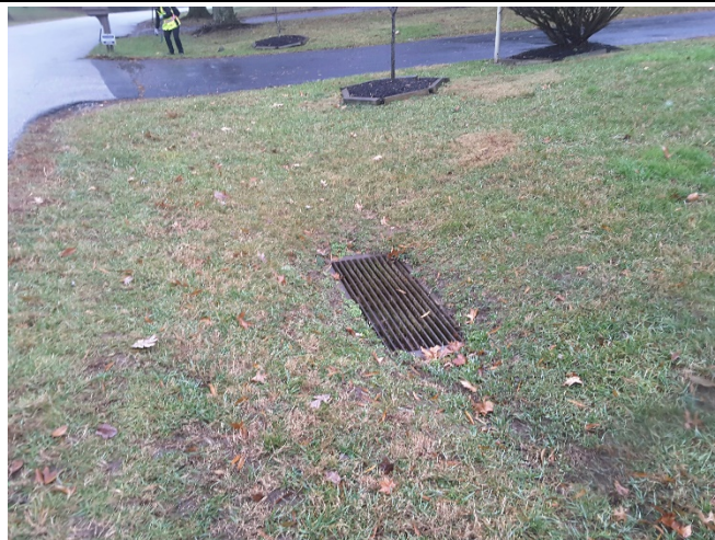
Figure 2: Typical inlet along MacAlpine Road.
