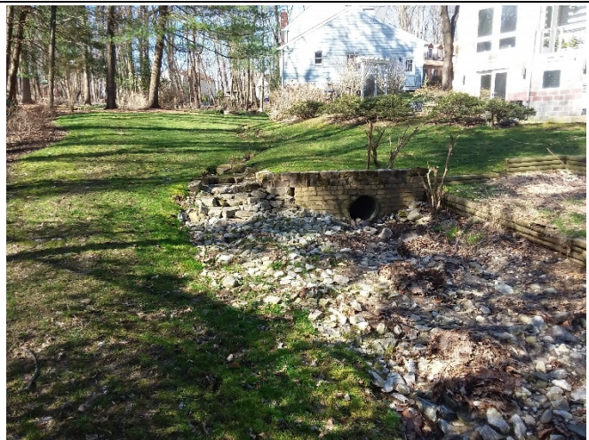
Figure 4: Opportunity to improve existing conveyance system.
