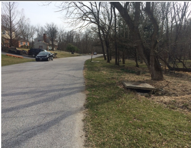
Figure 1: Opportunity to improve existing conveyance system.
