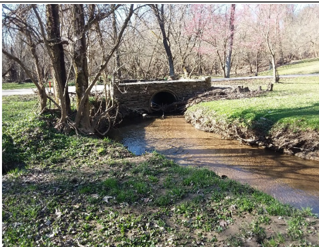
Figure 3: Opportunity to improve existing conveyance system.
