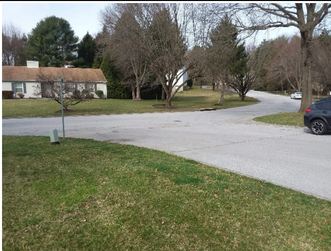
Figure 2: Opportunity to improve existing conveyance system.
