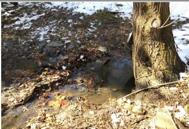
Figure 2: Storm drain outfall approximate location.
