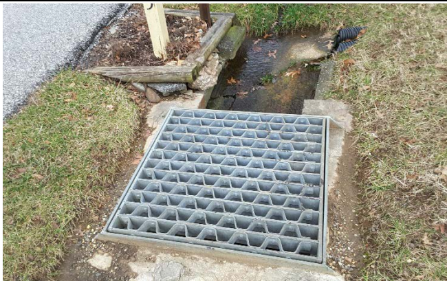
Figure 3: Typical inlet along MacAlpine Road.
