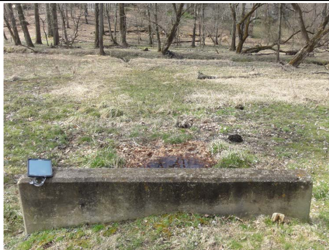
Figure 2: Opportunity to improve existing conveyance system.
