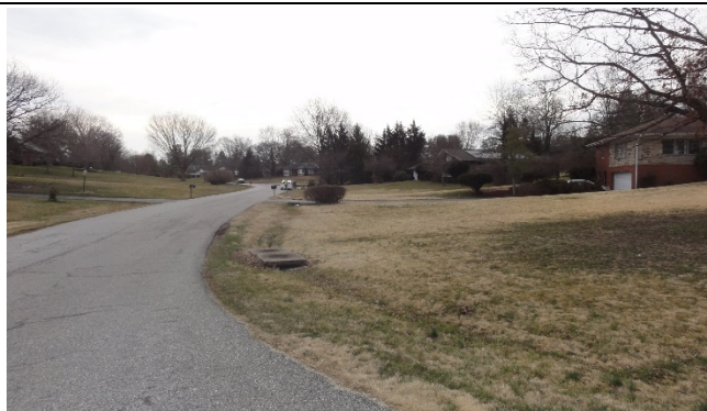
Figure 3: Opportunity to improve existing conveyance system.
