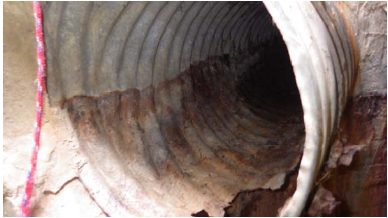
076.entry 1.station 8+44.manhole 3 21inch CMP inlet
