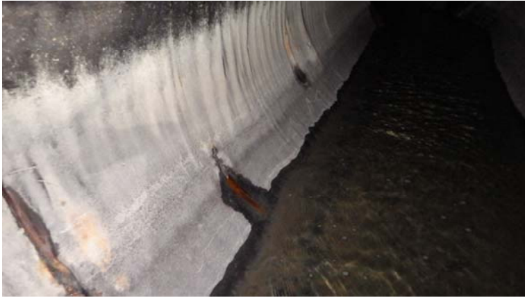
043.entry 1.station 4+00 infiltration continuous
