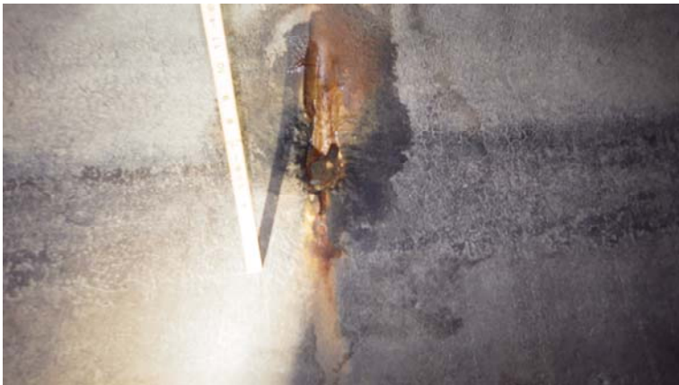
039.entry 1.station 3+14.pipe damage.soil water infiltration
