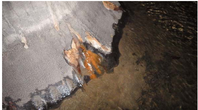
034.entry 1.station 1+97.infiltration
