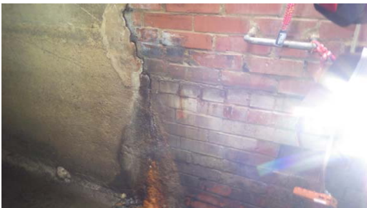
065.entry 1.station 7+17.manhole 4 fracture infiltration
