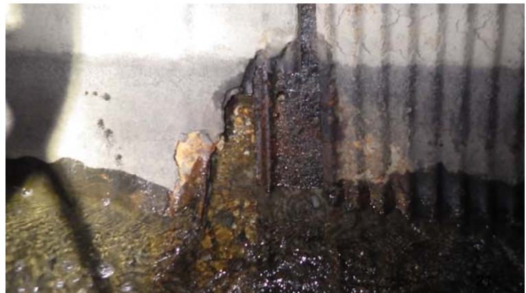
048.entry 1.station 4+33 joint damage soil water infiltration
