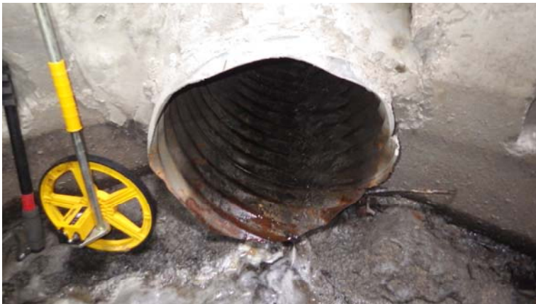
027.entry 1.station 1+19.24 inch CMP inlet
