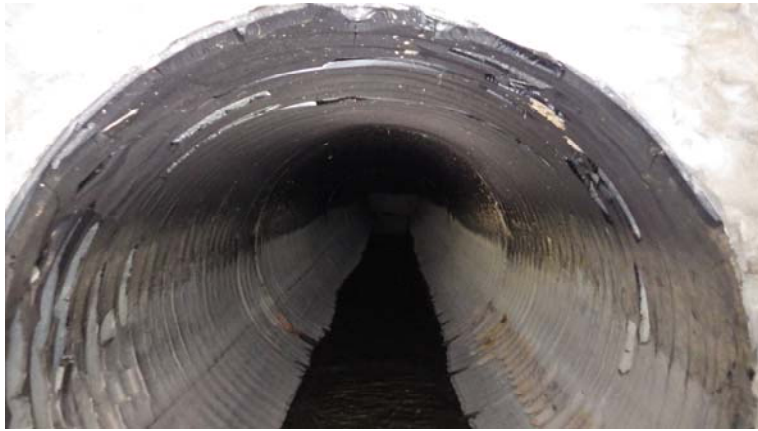
031.entry 1.station 1+19.84 inch CMP pipe
