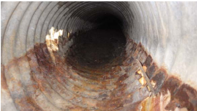
077.entry 1.station 8+44.manhole 3 21inch CMP inlet
