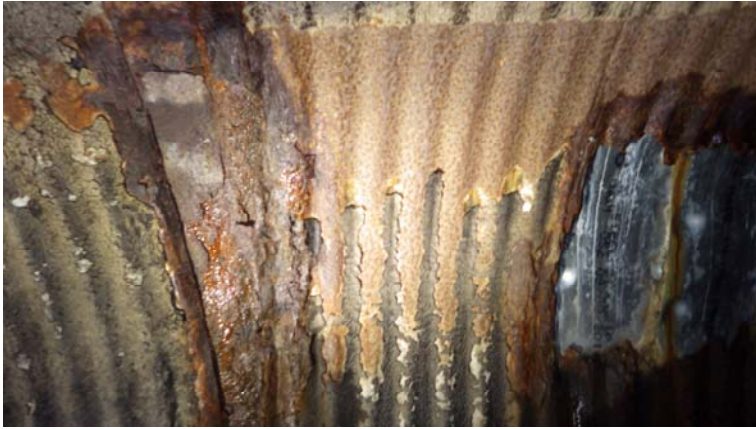
049.entry 1.station 4+40.pipe damage corrosion
