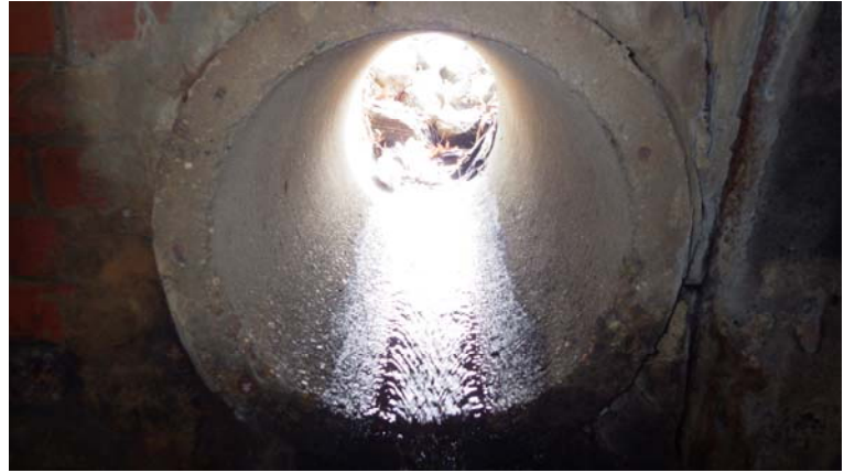
062.entry 1.station 7+12.15 inch RCP inlet
