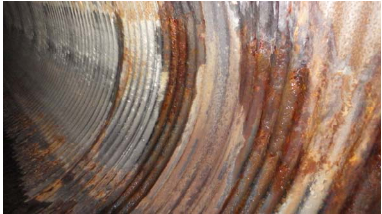
052.entry 1.station 4+40.pipe damage corrosion
