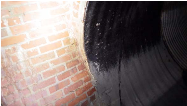
045.entry 1.station 4+26 masonry manhole structure
