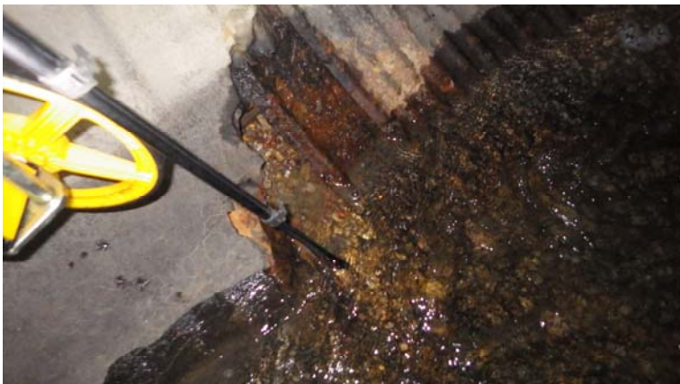
047.entry 1.station 4+33 joint damage soil water infiltration
