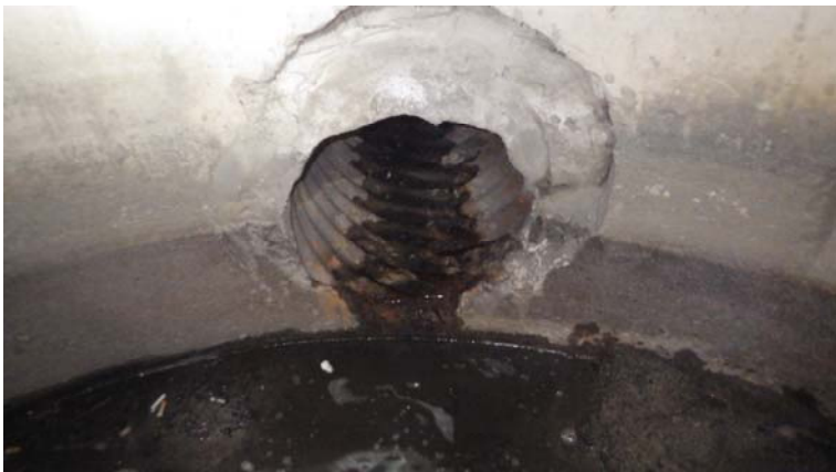
029.entry 1.station 1+19.18 inch CMP inlet
