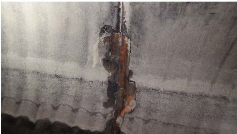
041.entry 1.station 3+59.pipe damage
