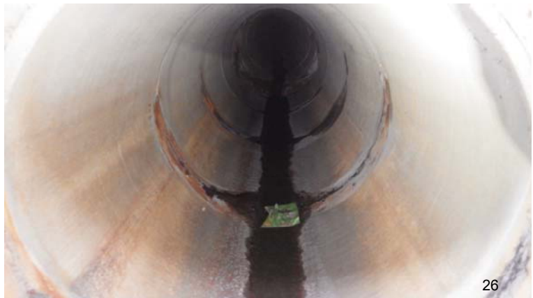
078.entry 1.station 8+44.manhole 3 east 42 inch RCP inlet
