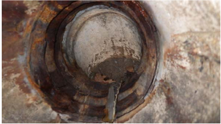
068.entry 1.station 7+75.10 CMP inlet at 1200
