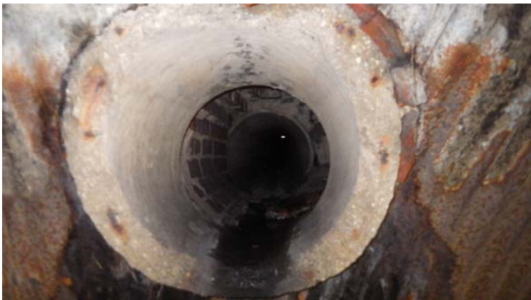
053.entry 1.station 4+43.15 inch RCP inlet
