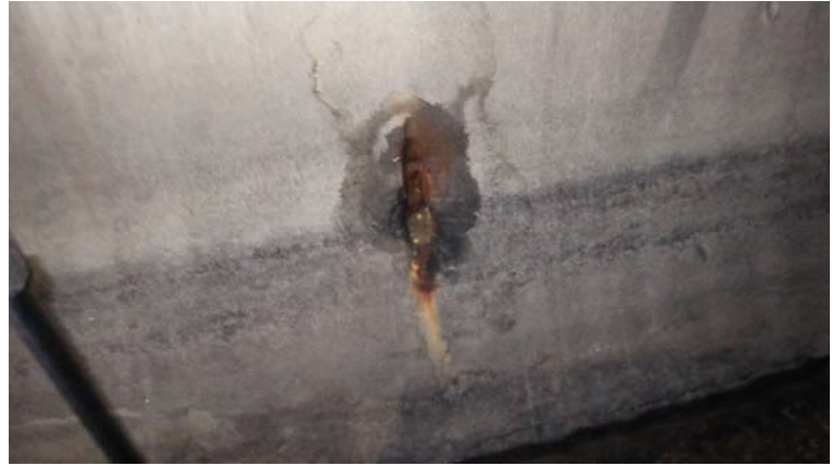
038.entry 1.station 3+14.pipe damage.soil water infiltration
