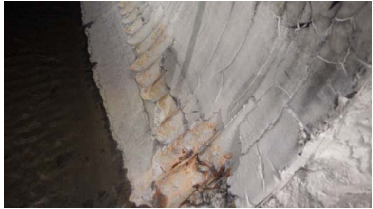
032.entry 1.station 1+22.loss of protective material.corrosion
