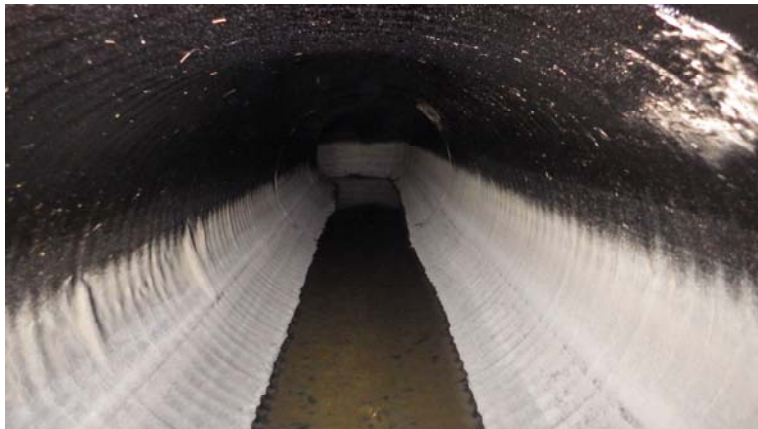
033.entry 1.station 1 +60.pipe deformity
