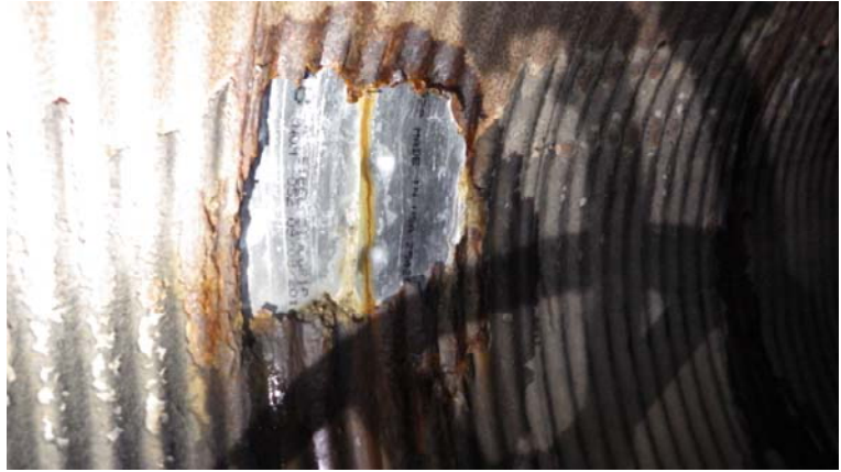
050.entry 1.station 4+40.pipe damage corrosion
