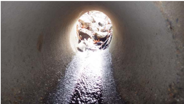
063.entry 1.station 7+12.15 inch RCP inlet
