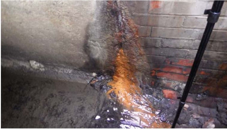
067.entry 1.station 7+17.manhole 4 fracture infiltration
