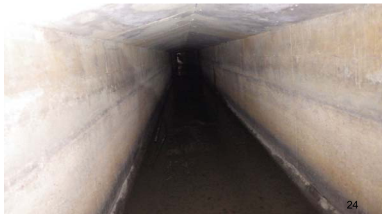
066.entry 1.station 7+17.6 x 6 box culvert
