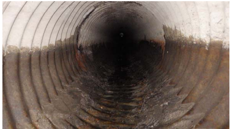
028.entry 1.station 1+19.24 inch CMP inlet pipe
