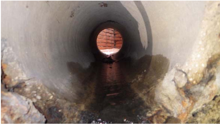
057.entry 1.station 6+68.15 inch RCP inlet
