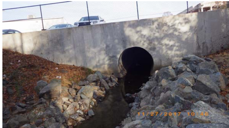
022.downstream headwall
