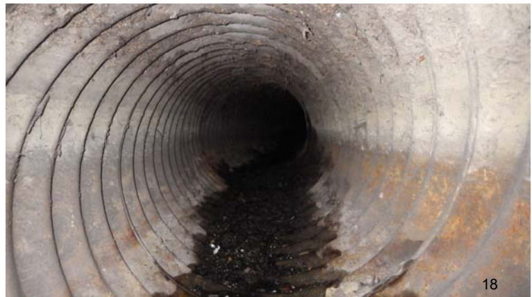
030.entry 1.station 1+19.18 inch CMP inlet pipe
