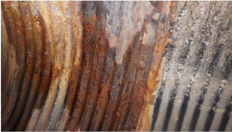
051.entry 1.station 4+40.pipe damage corrosion
