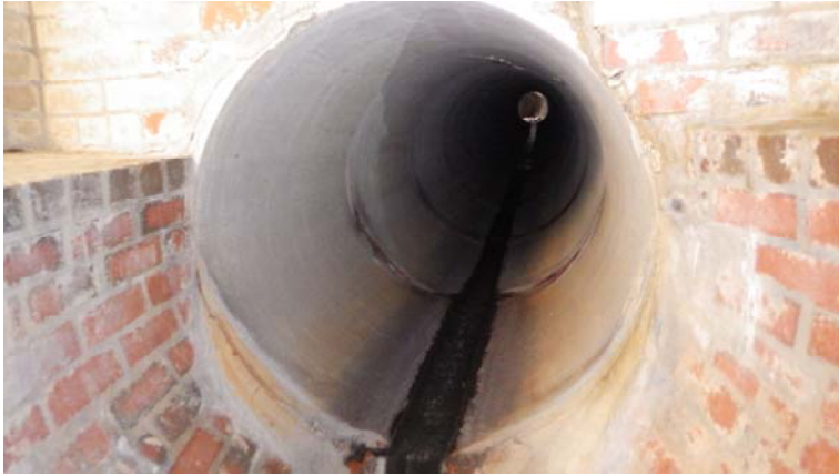
073.entry 1.station 8+44.manhole 3 42 inch RCP inlet
