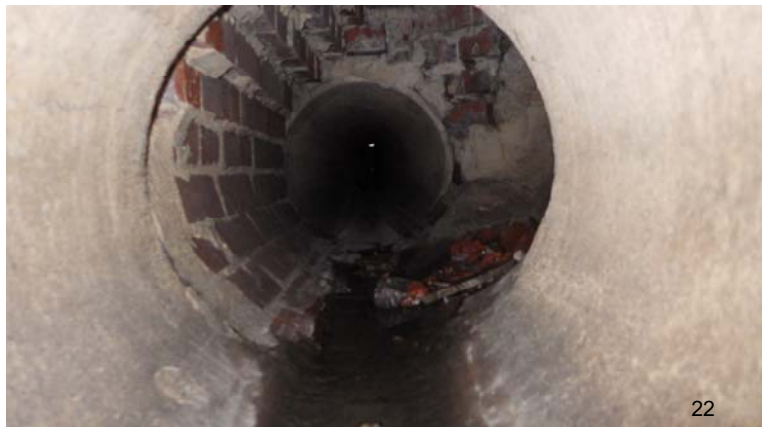
054.entry 1.station 4+43.15 inch RCP inlet
