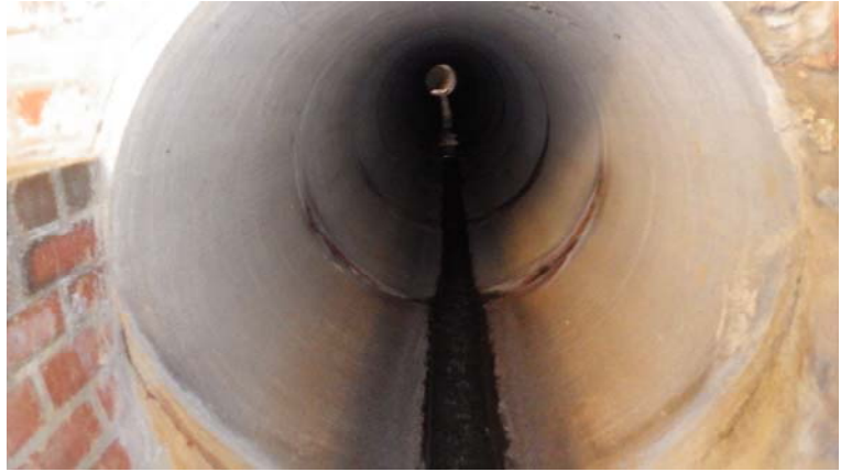
074.entry 1.station 8+44.manhole 3 42 inch RCP inlet
