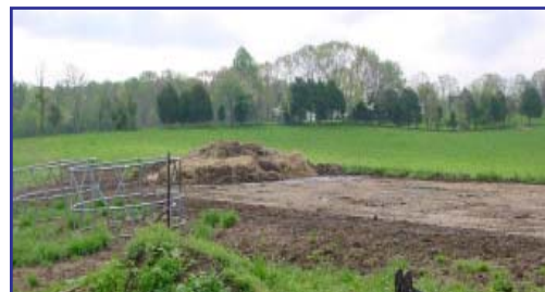
Stabilize heavy use areas with geotextile fabric and rock. 1
