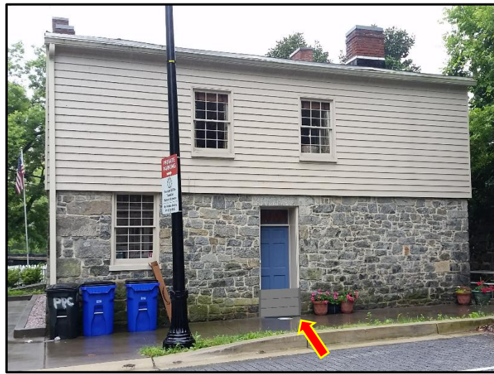
Rendering of Stoplog Door Closure Panel
