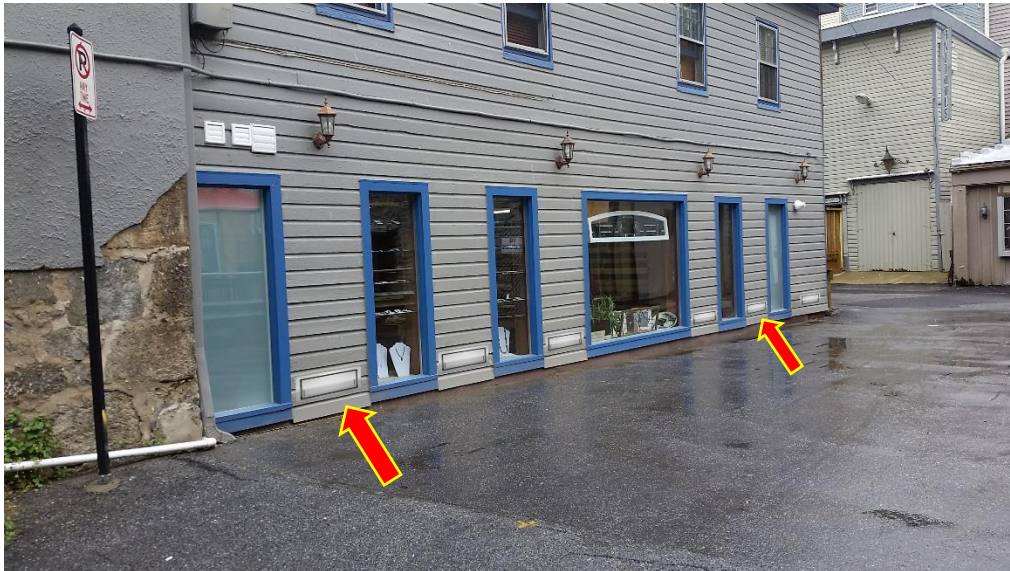
Rendering of Wet Flood Proofing Louvers/Openings
