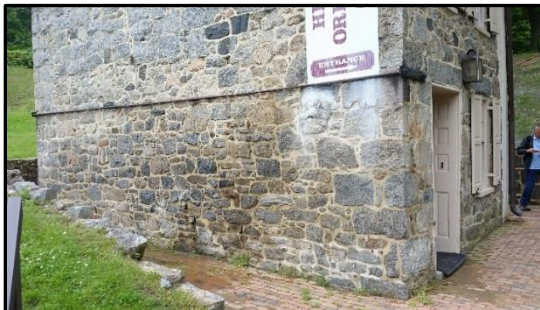
3. East Elevation, Stone foundation and exterior wall
