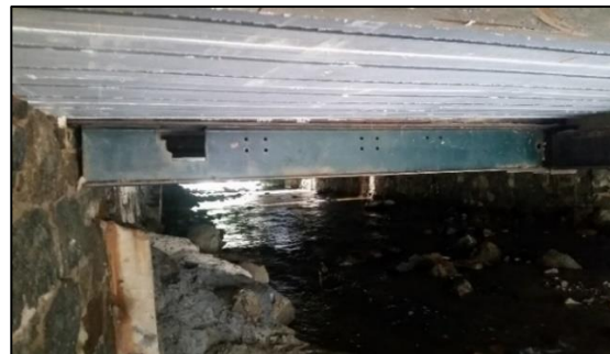
4. Extraneous steel framing below first floor slab
