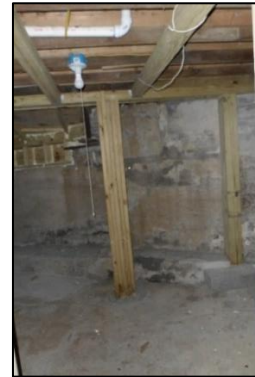
4. Basement with supplemental wood framing
