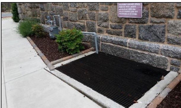
3. At-grade access grate on west elevation
