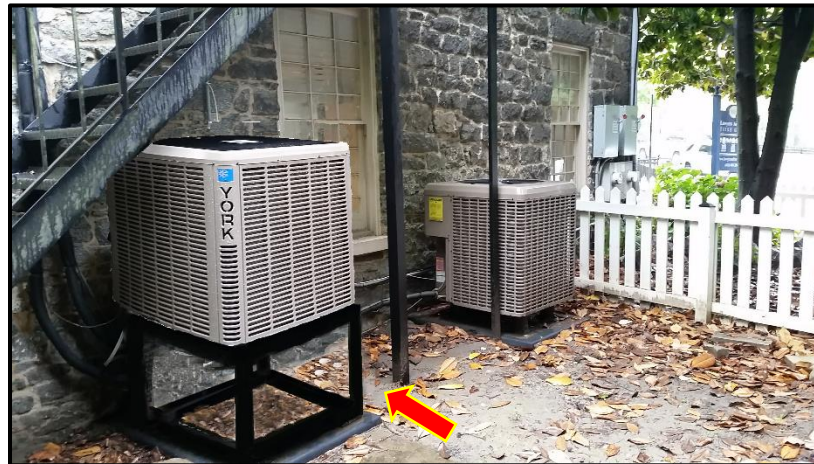
Rendering of Elevated External Utilities (HVAC unit on the left is elevated)
