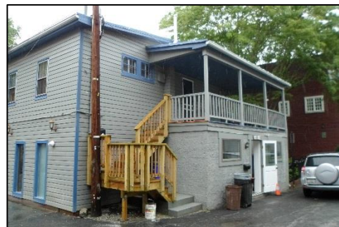
4. Small CMU addition on south elevation
