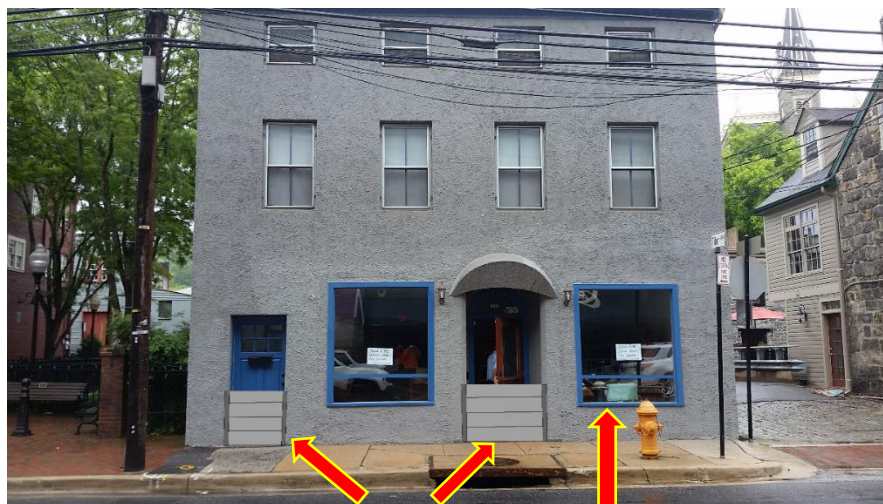
Rendering of Stoplog Door Closures and Structural Windows
