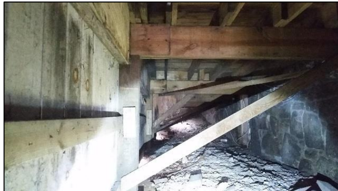
4. Porch framing in basement area
