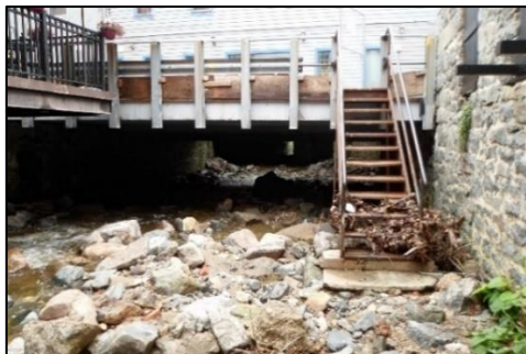
3. Metal access stair reducing stream conveyance
