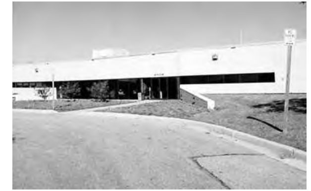
Howard County Detention Center
